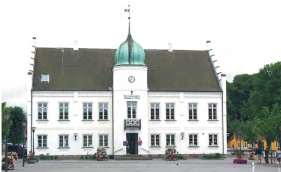
Just a few minutes from the new cultural centre you will find the old town hall
